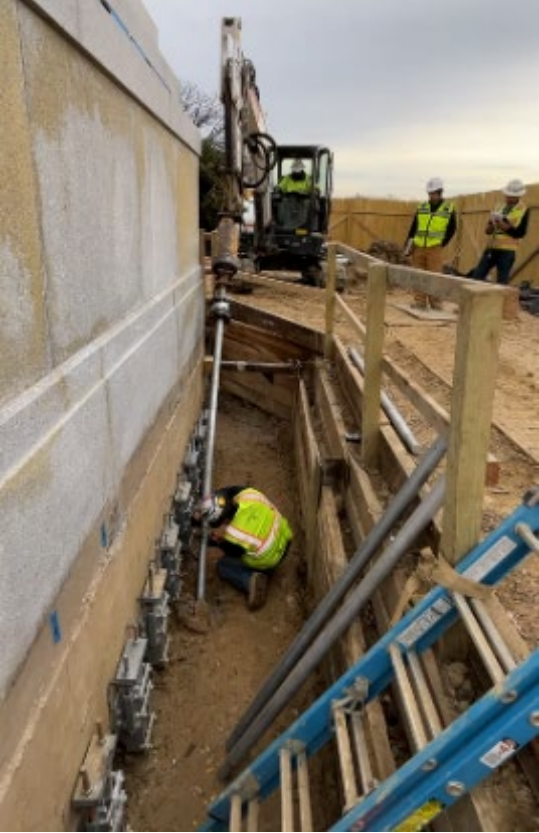
Helical Anchor Installation
