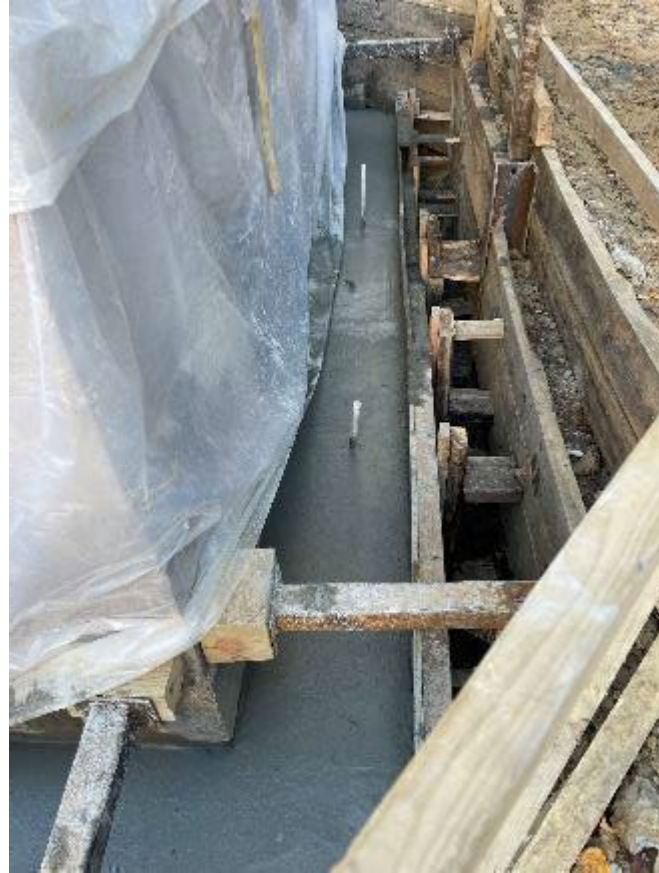
Placed Grade Beam with High Pressure Grout Ports
