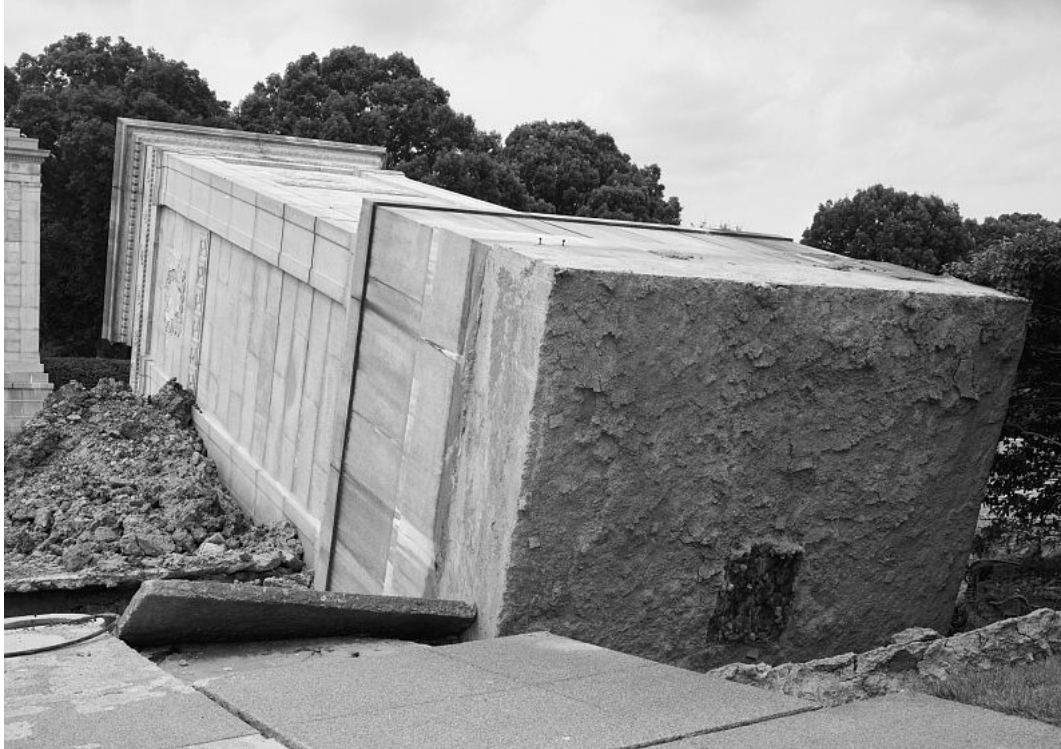
July 1996, Pylon 2 toppled due to the excavation of a utility trench
