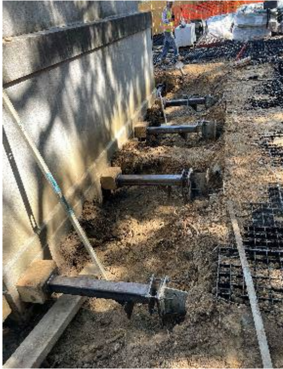
H Piles & Support Beams
