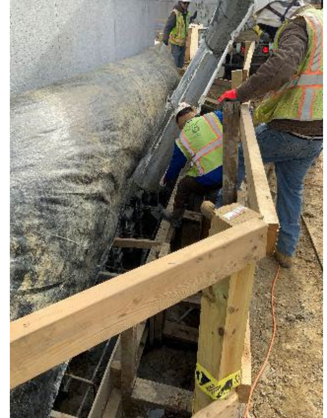
Concrete Grade Beam Placement
