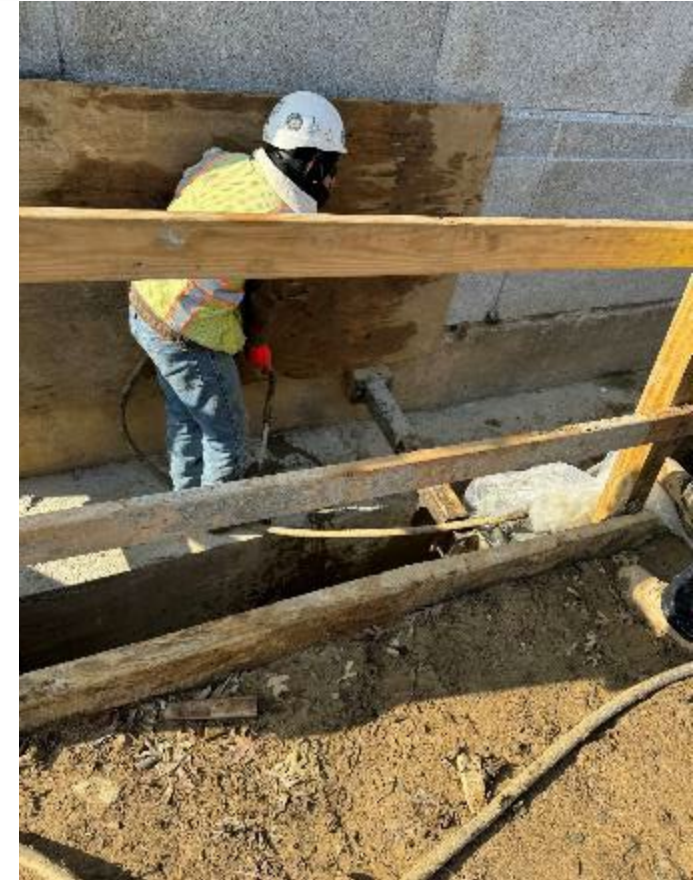
High Pressure Grout Placement
