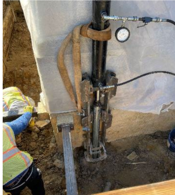
Support Bracket and First Push Pier
