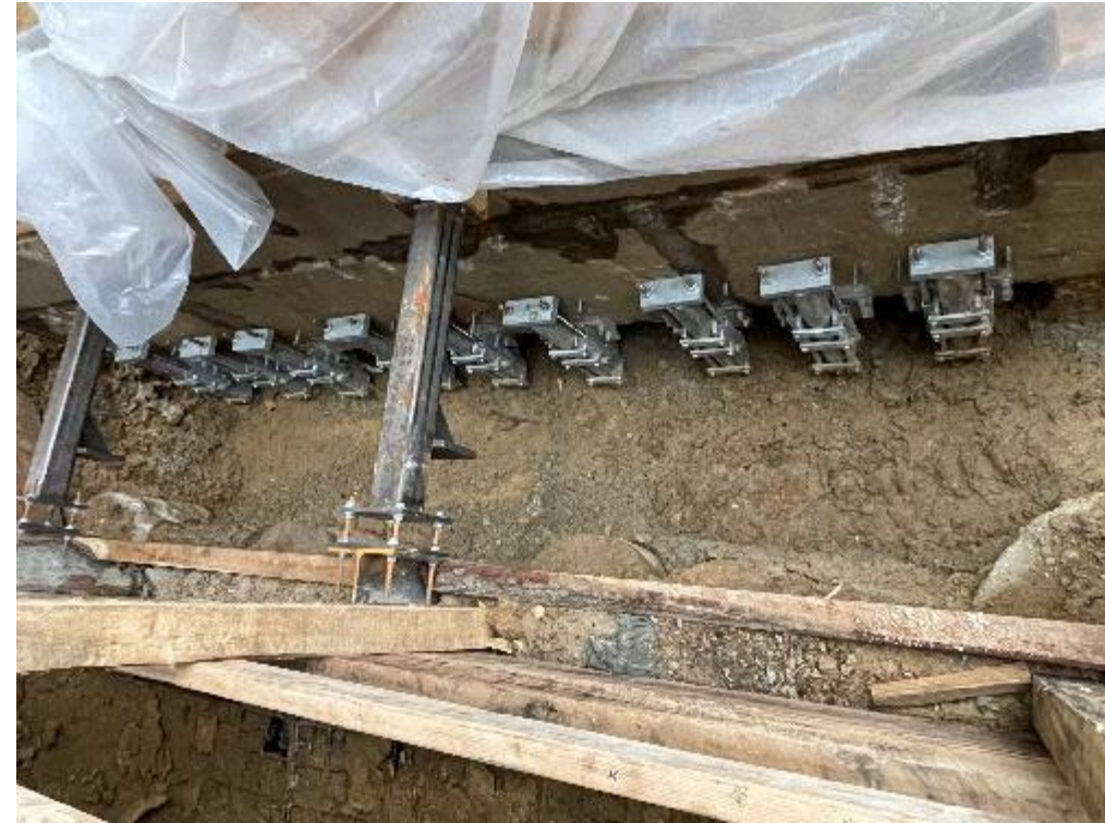
Completed Support Bracket Installation
