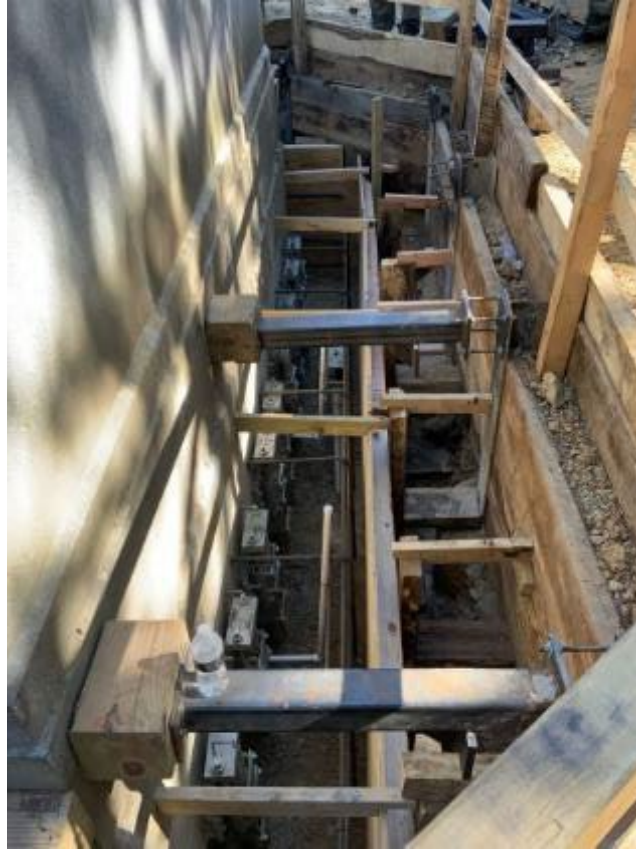
Concrete Grade Beam Reinforcement
