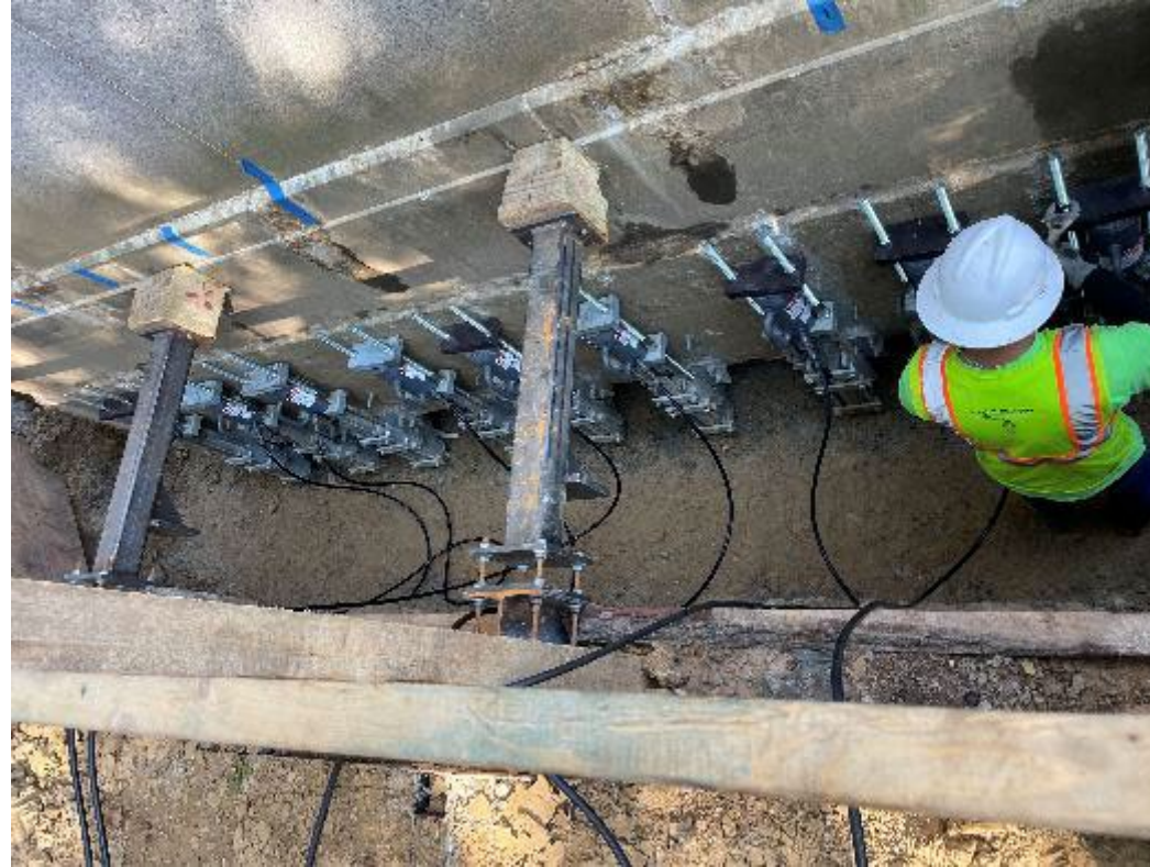
Use of Hydraulics for Lifting
