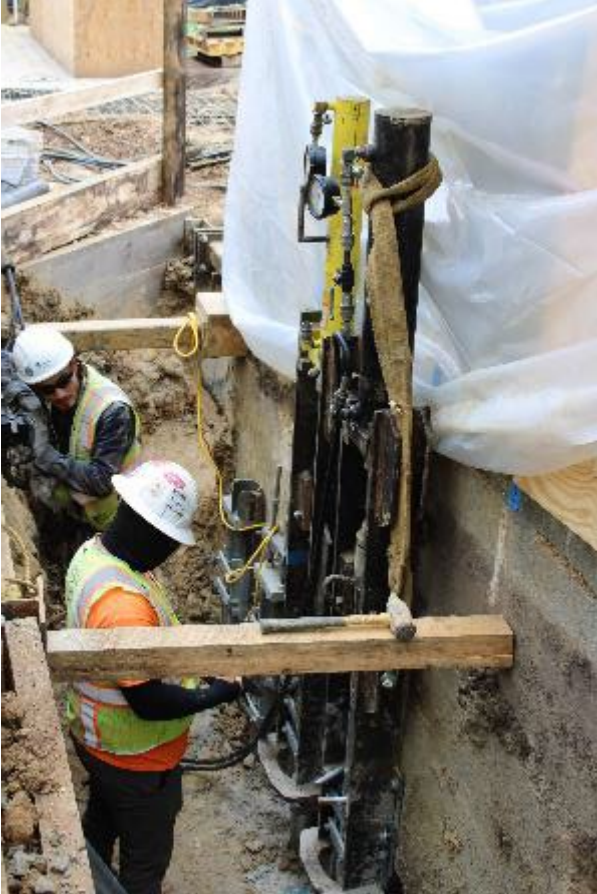
Push Pier Installation
